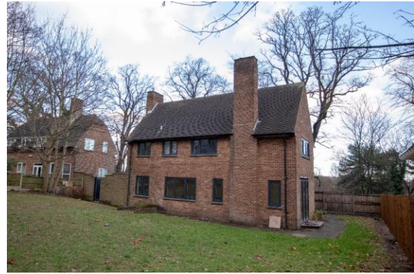
Figure 4: Back view of test building
