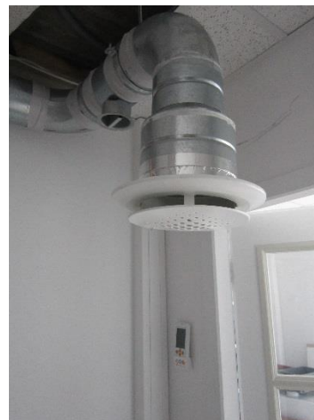
Figure 1: Pictures of the Positive Input Ventilation in the experimental house – Left: Central ventilation device in the attic, Right: Air diffusing unit in the first floor hall
