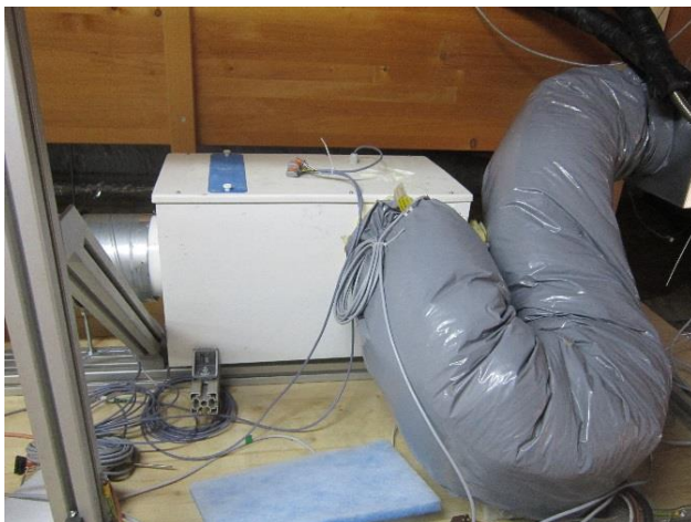
Figure 1: Pictures of the Positive Input Ventilation in the experimental house – Left: Central ventilation device in the attic, Right: Air diffusing unit in the first floor hall
