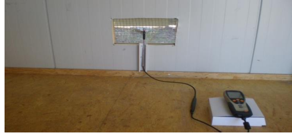
Figure 6b: Measurements point at ventilation inlet
