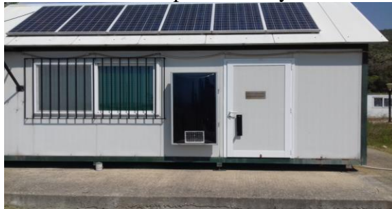
Figure 2: Solar air collector
