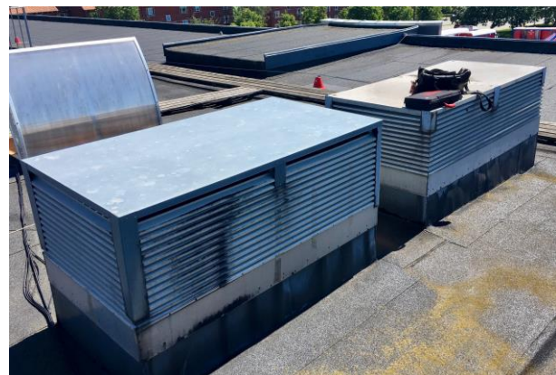
Figures 12 and 13: Fresh air intake problems. On the left, Fig. 12, an example of a blocked fresh air inlet grille.
