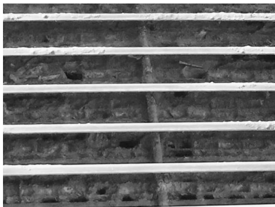
Figures 12 and 13: Fresh air intake problems. On the left, Fig. 12, an example of a blocked fresh air inlet grille.
