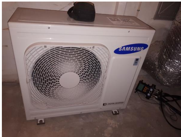
approx. 4.000 m 3 /h, but no-one was sure which areas in the building were actually supplied by this system. Figures 16 and 17: Consequences of alteration problems: Some offices that are no longer supplied with air from the ventilation unit (Fig. 14 and 15) are overheating, but because the tenants just think that the ventilation system is inadequate (instead of just not being connected) they install split air conditioners (Fig. 16, left photo) adding to the energy burden, at the same time as the ventilation system is running inefficiently and is underused. The photo on the right, Fig. 17, shows a small server room with ventilation connected to the system shown in figure 14. It needs ventilation constantly, 150 m 3 /h 168 hours/week, but it is connected to the same system supplying
